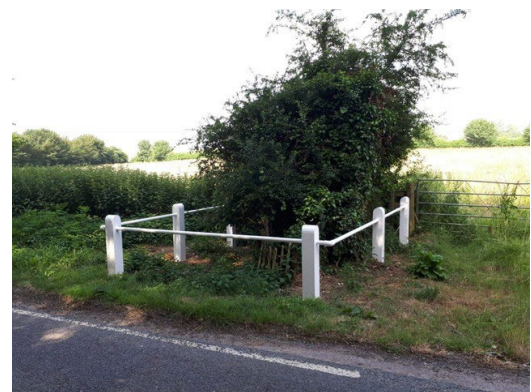
Hempstead railings- after
